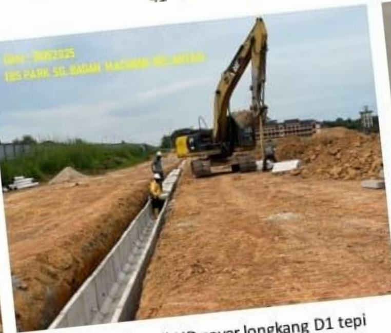
Roadwork: Lay c/run for road base sebelah petak 41 - 38
